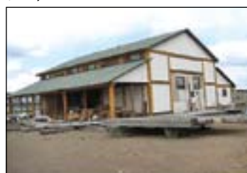
2 ACRES BUILDING ACCOMMODATES MANY USES
