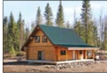
PINE LOG HOME - READY TO FINISH
