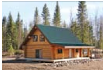
PINE LOG HOME - READY TO FINISH
