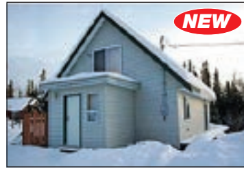
READY TO FINISH!
