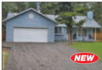
THE GARAGE IS BACK AND THE ROOF IS NEW!
